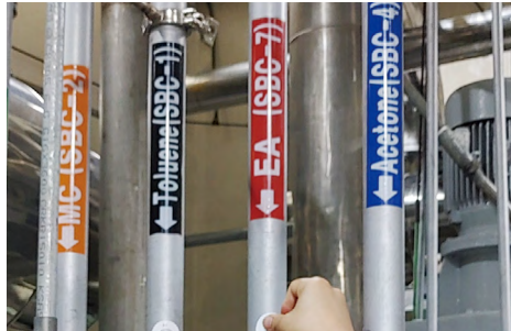
Labeling of hazardous chemical pipelines
